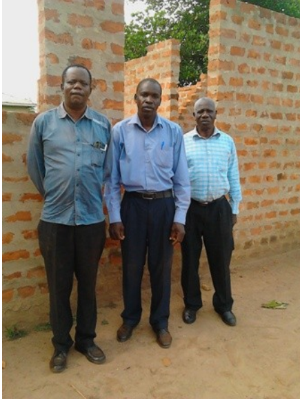
The new house for the pastor that need to be roofed
